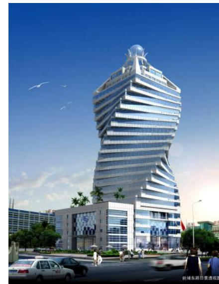
Ruihua Technology Building, Xiamen, China
