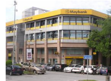
Maybank Damansara Utama, Malaysia
