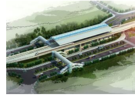
Guangzhou Metro 6 line, Guangdong, China
